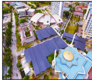
Solar carpark system
